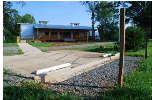
Rain garden and level spreader installed to control stormwater at Yesterday Spaces Event Center and Farm
