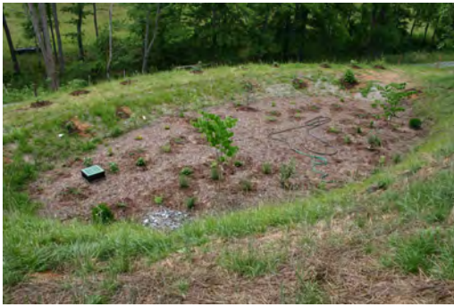
Rain garden and level spreader installed to control stormwater at Yesterday Spaces Event Center and Farm
