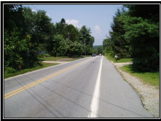
SR 1224 Northbound Approach
