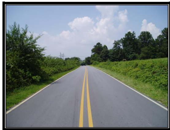
SR 1238 Westbound Approach
