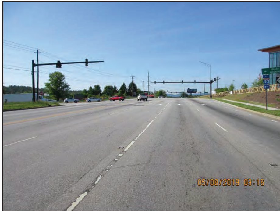
Westbound Approach looking West
