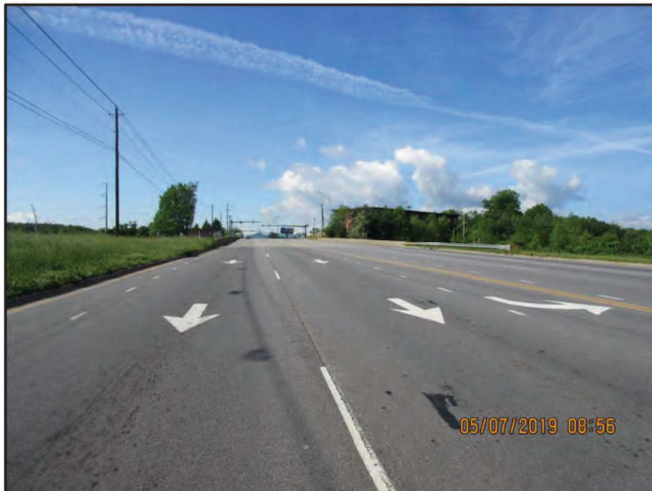
Eastbound Approach looking West
