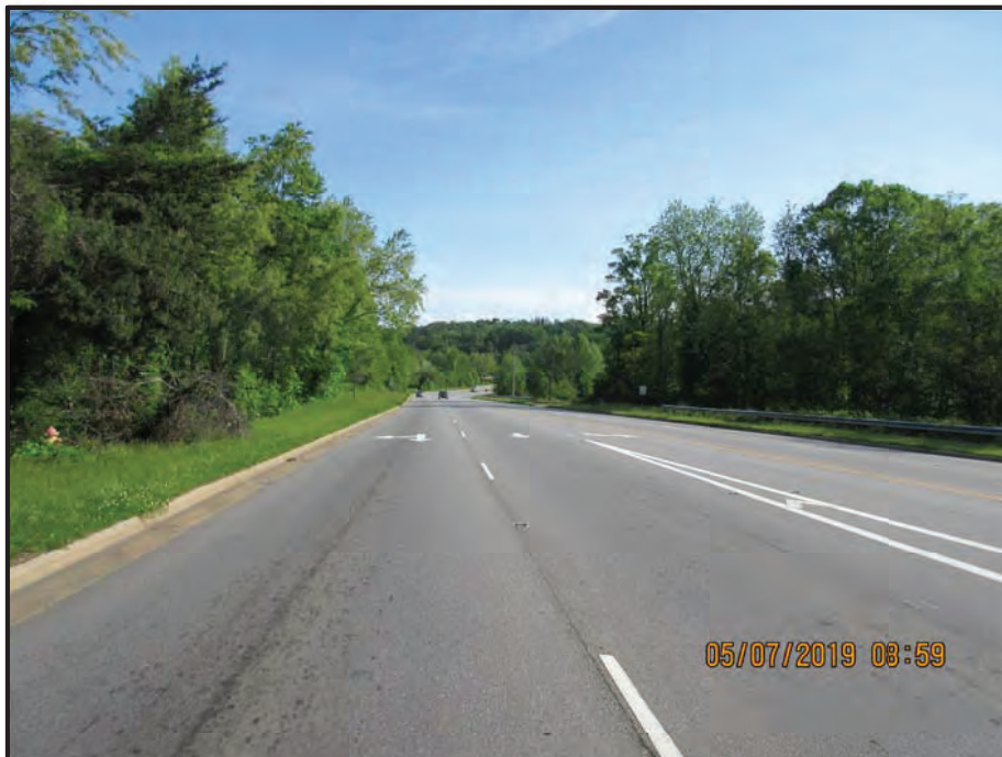
Westbound Approach looking East
