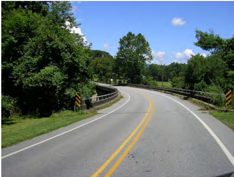
SR 3413 (South Bear Creek Road) looking northbound toward the bridge over I-240
