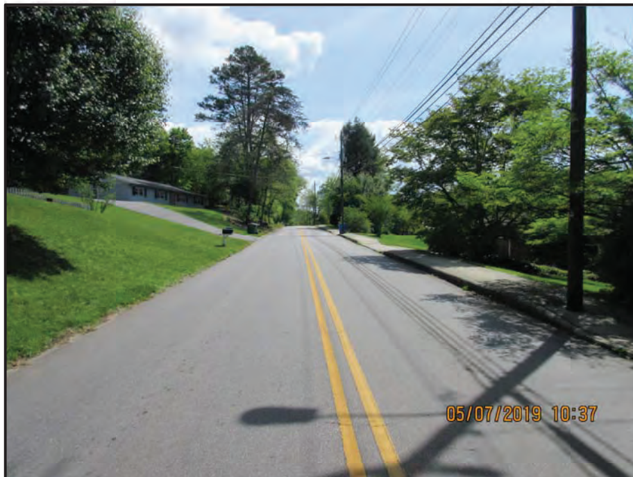
Northbound Approach looking South
