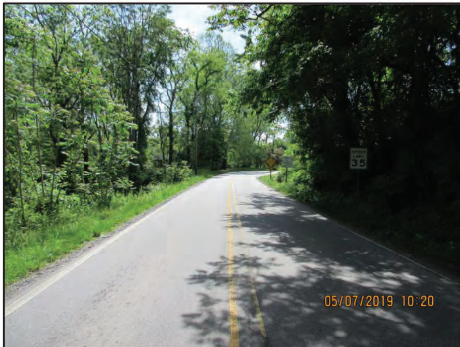
Northbound Approach looking South
