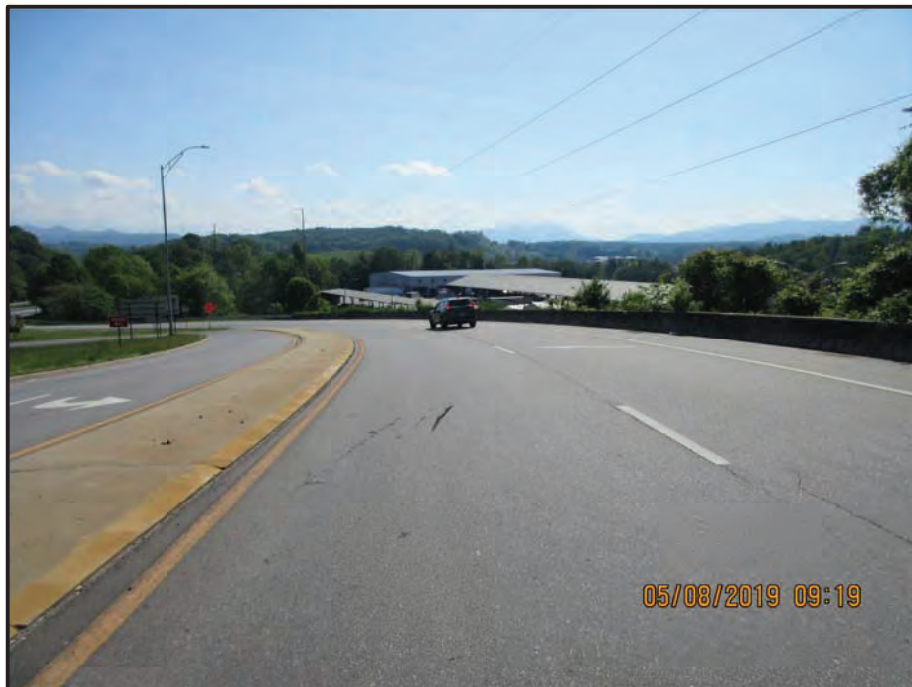
Northbound Approach looking South
