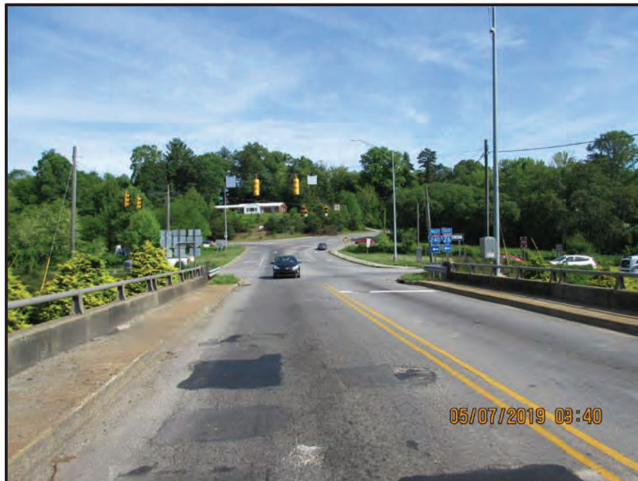
Westbound Approach looking East
