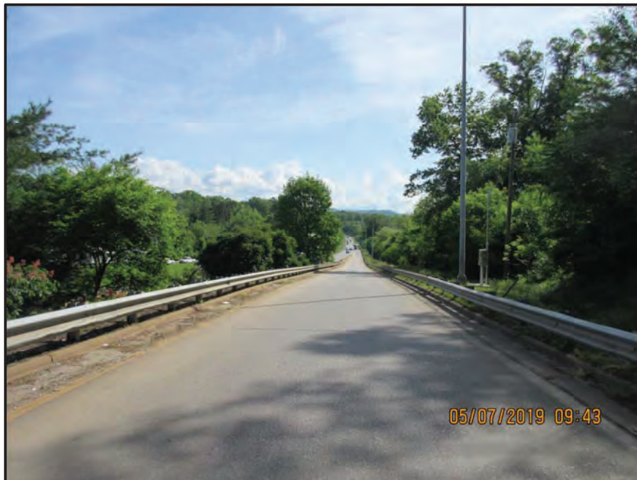
Northbound Approach looking South
