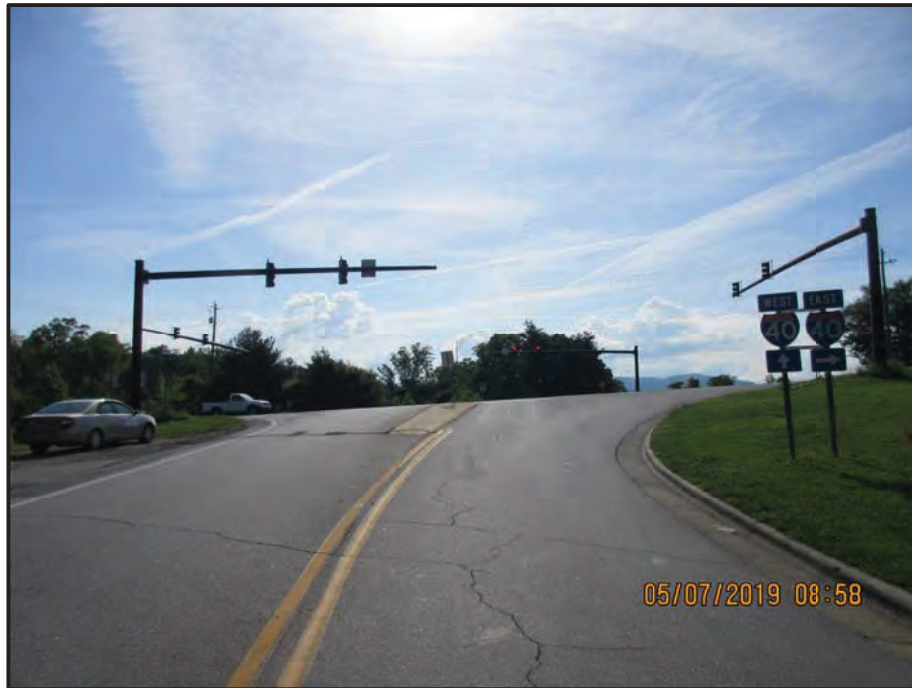
Southbound Approach looking South
