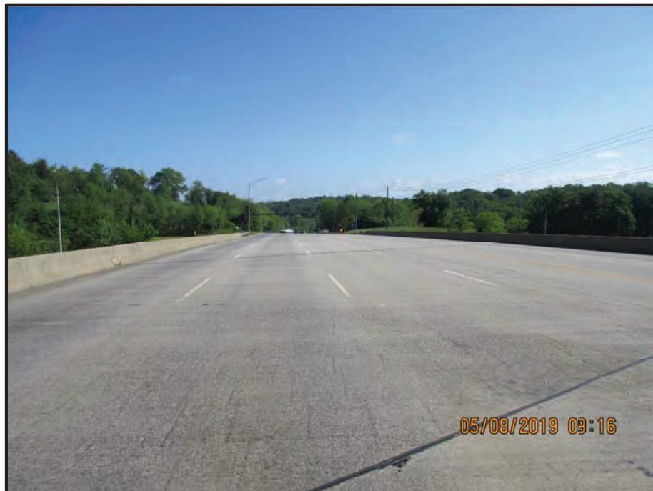
Westbound Approach looking East
