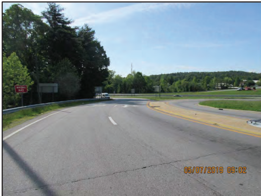
Northbound Approach looking South
