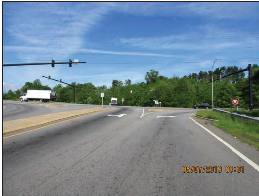
Northbound Approach looking North
