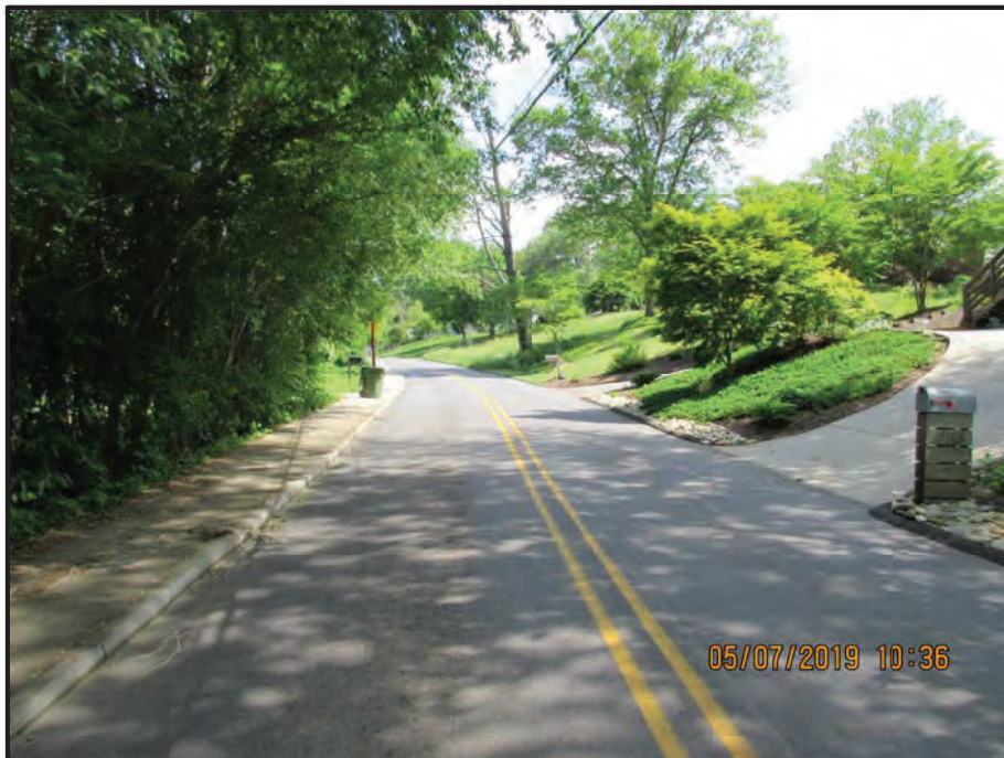
Westbound Approach looking East
