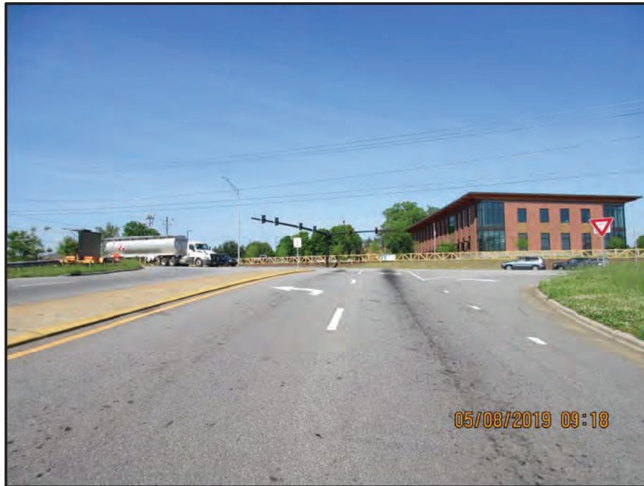
Northbound Approach looking North
