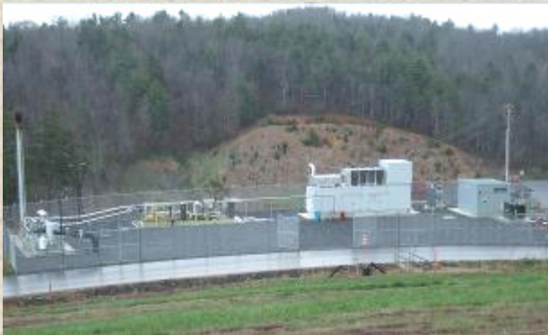
Landfill Gas to Energy Facility
