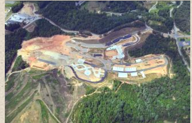
Aerial View of the Public Safety Training Center
