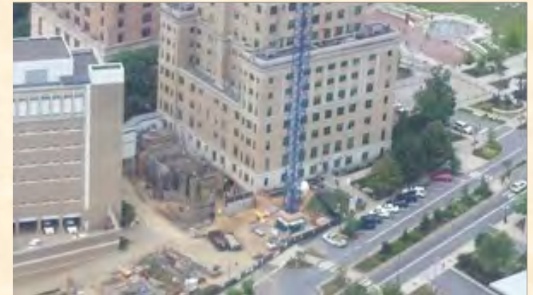
Courthouse Life Safety Tower Construction
