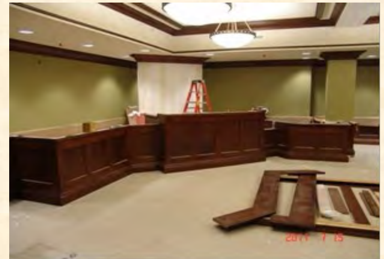
Renovations to courtrooms
