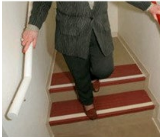
Contrasting color on steps can help with visibility.
