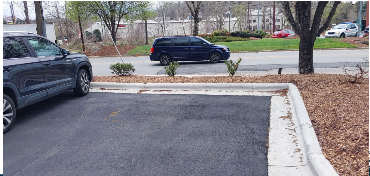
Bore pit in parking lot of Eurosport Asheville (top & bottom photos)
