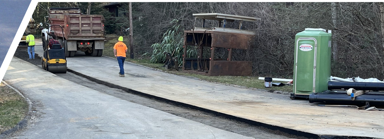
Installing 6" asphalt binder course per COA street standards
