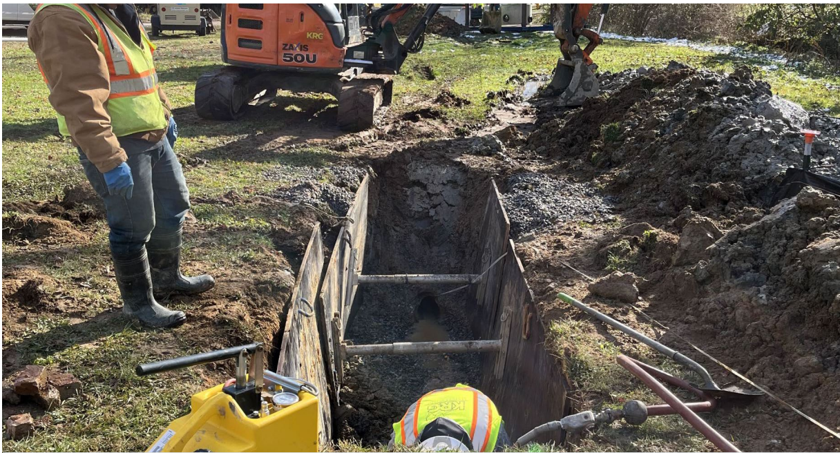
Pipe bursting bore pit (top left); bursting head and HDPE pipe (top right); winch machine (lower left); bursting head entering old manhole (lower right)
