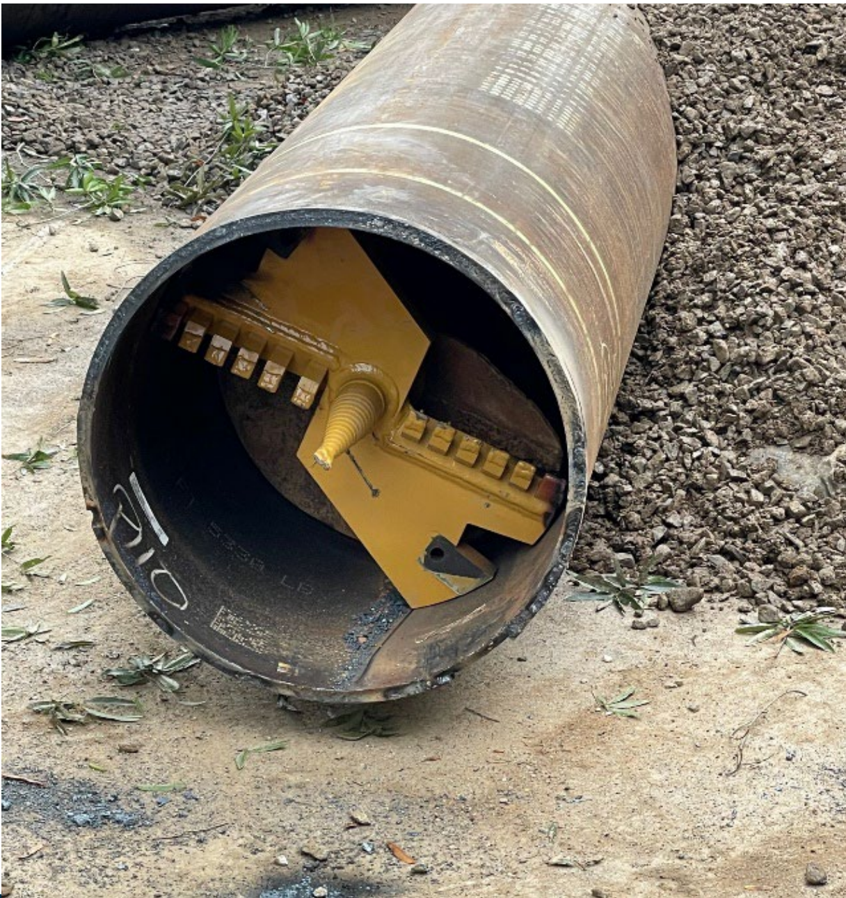
24" jack and bore auger inside steel casing pipe
