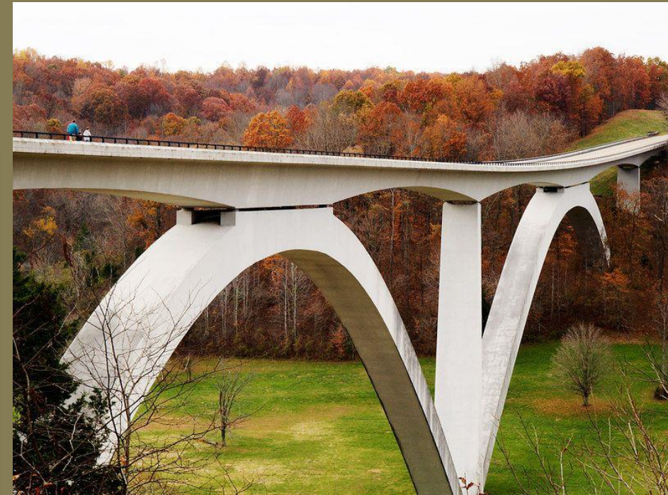
Example: Natchez Trace Parkway Bridge
