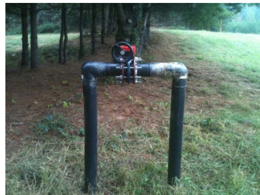
Gas Valve at Area A Buncombe County Closed Landfill
