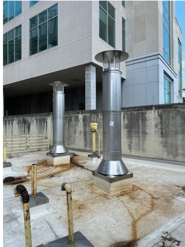
Detention Center Repairs
