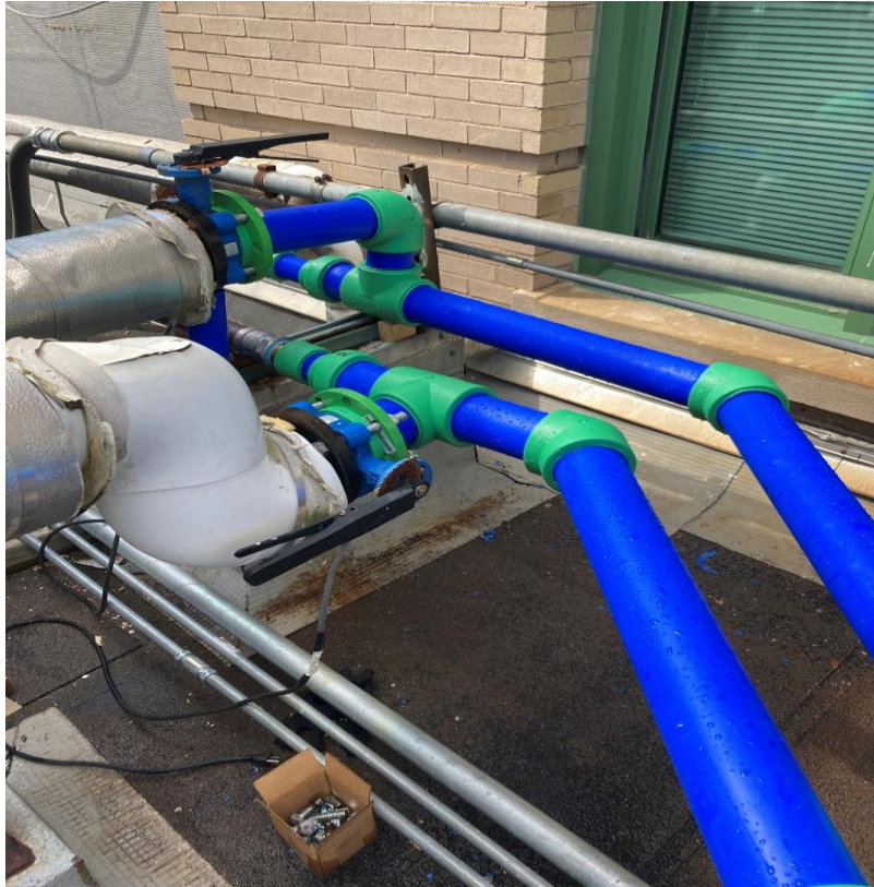
County Courthouse Repairs
