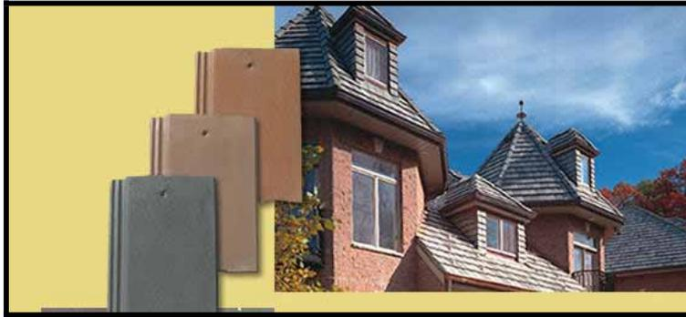
**Wood Shakes:** Wood shakes differ from wood shingles in two ways; they are much thicker than wood shingles and less uniform in shape and size. Wood shakes may be hand split. They are attached to the roof by nails.
