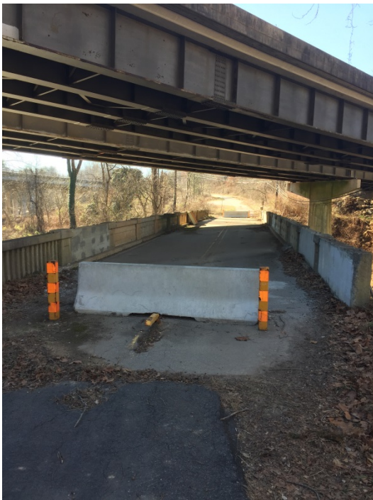
Buncombe County Bridge #216 is an existing historic bridge over Hominy Creek and under I-40.
