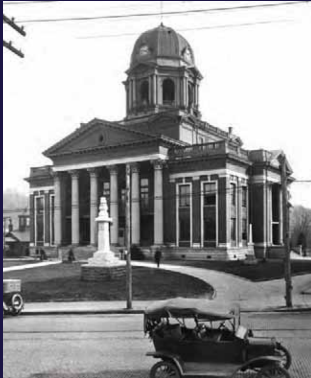
The Union County Courthouse on College Street in 1903
