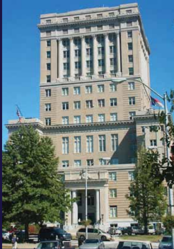
The Buncombe County Courthouse as it stands today
