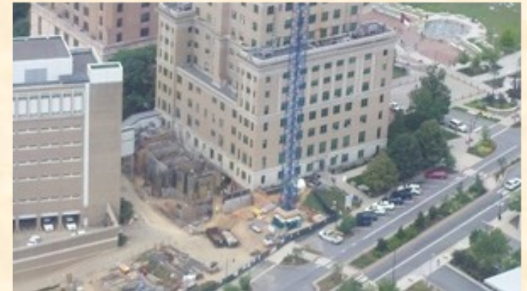
Courthouse Life Safety Tower Construction
