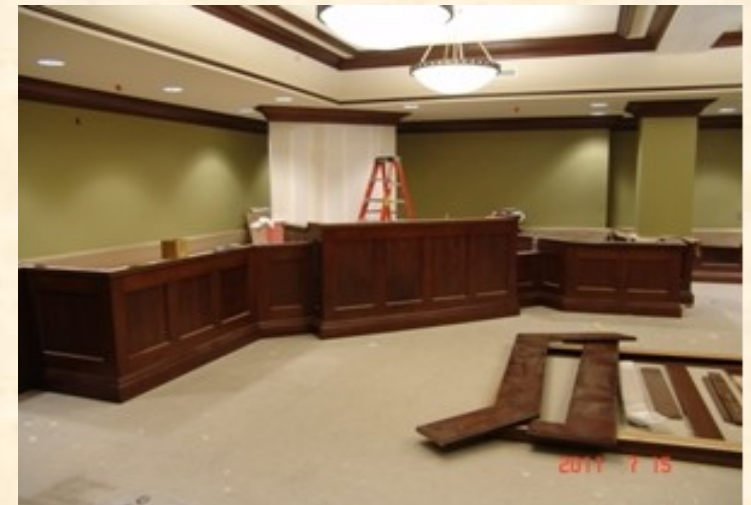
Renovations to courtrooms
