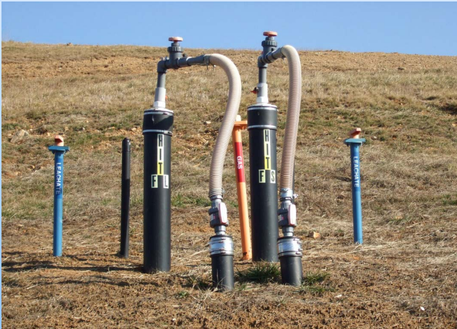
Leachate Injection and Gas Recovery System
