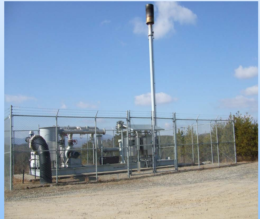
Methane Flare Station Reduces Greenhouse Gas Emissions
