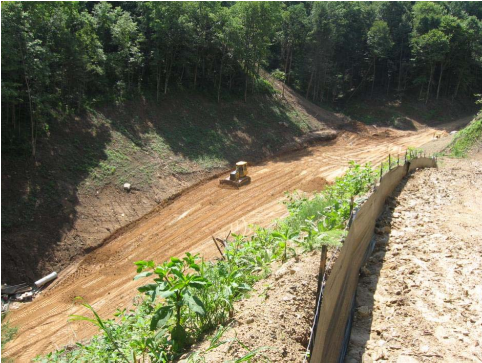
POND 13 CONSTRUCTION FOR PHASE 5 C&D LF
