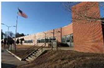
ADMINISTRATIVE SERVICES BUILDING Switchgear Replacement
