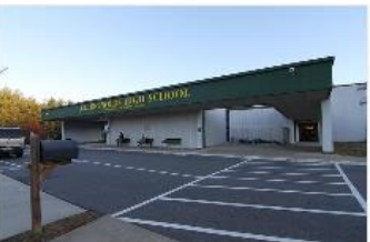
A.C. REYNOLDS HIGH Roofing Projects
