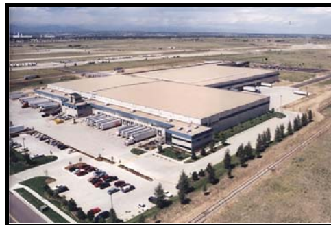
Cold Storage Warehouse
