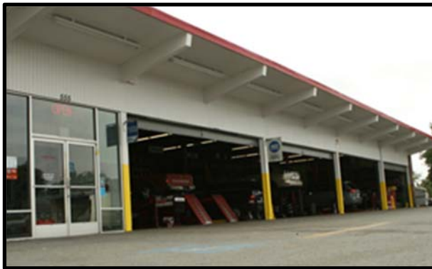
Auto Service Garage
