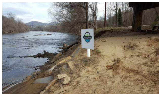
River Bank Beneath Pearson Bridge Road
