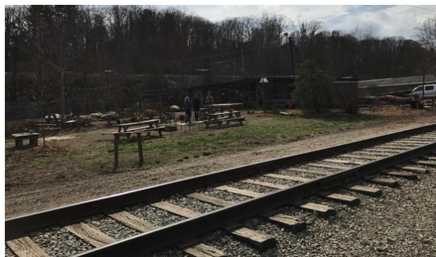
Existing Rail Line
