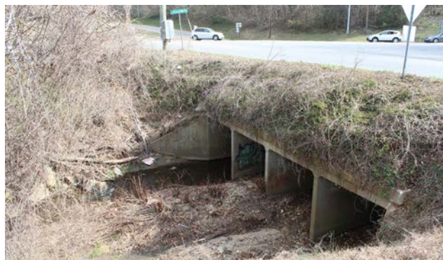
Culvert Under Riverside Drive
