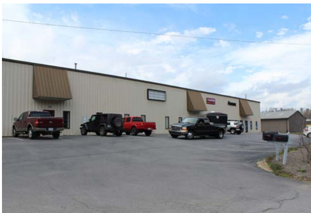
Businesses on Riverside Drive
