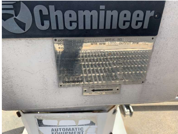
Figure 2-8. Flocculator motor
