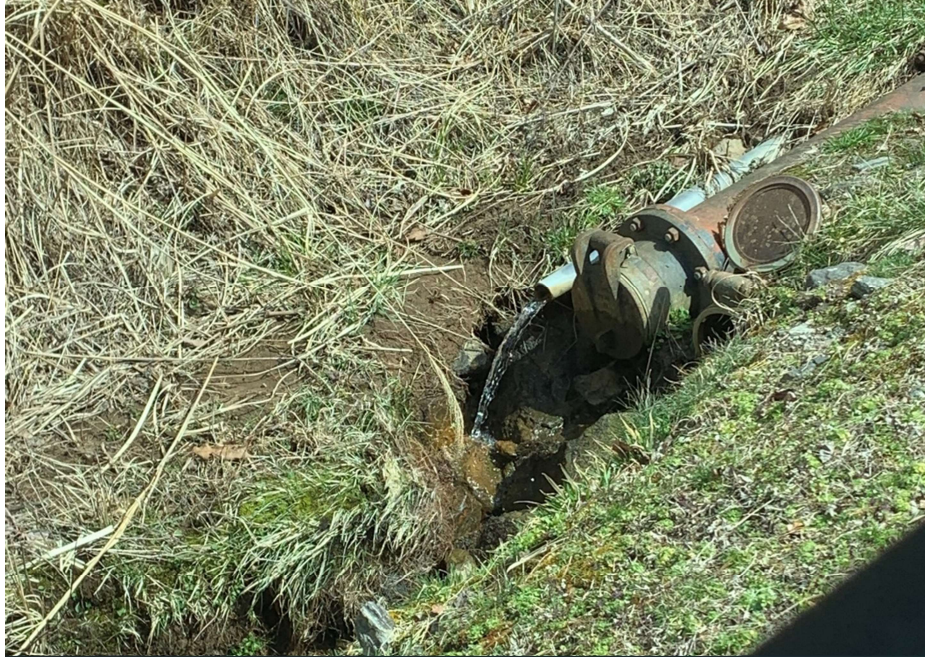
Figure 2-22. NPDES Discharge pipe into drainage ditch
