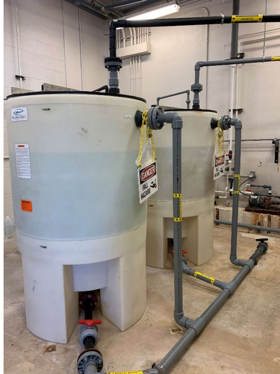
Figure 2-19 Alum and caustic day tanks
