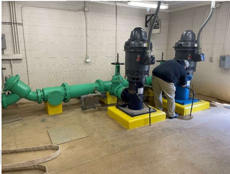
Figure 2-1 Vertical turbine pumps
