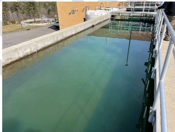
Figure 2-9. Northside Sedimentation Basin
