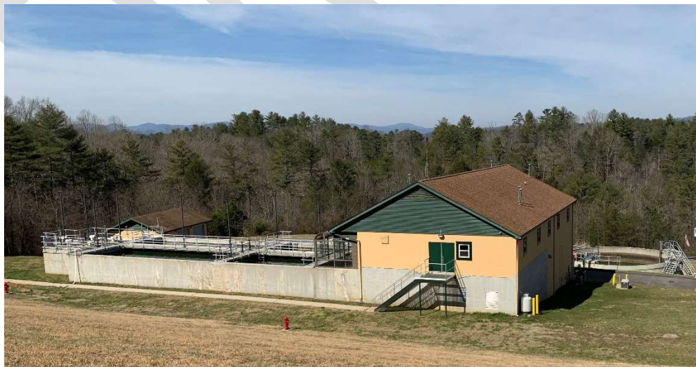
Figure 2-20. WTP building, picture facing north.
