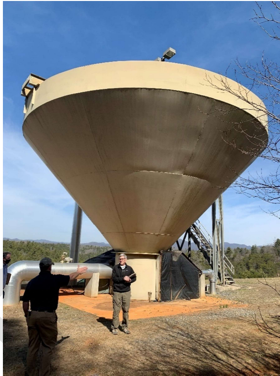
Figure 2-4. Existing Claricone
