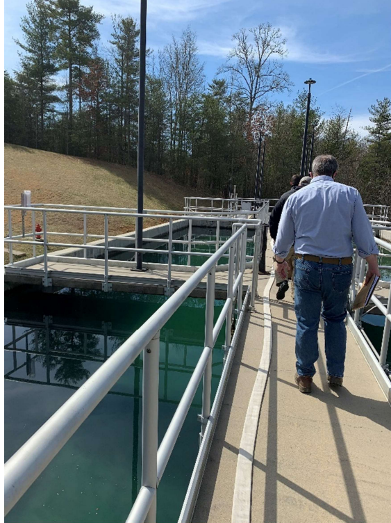
Figure 2-10. Walkway between sedimentation basins
