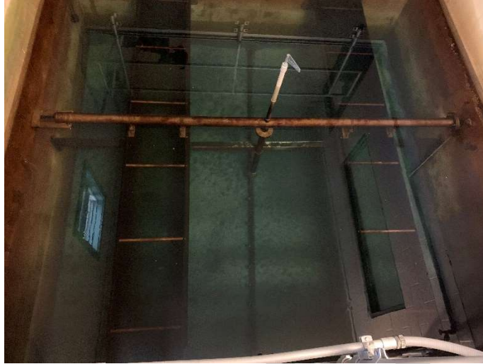
Figure 2-12 Top of media filter
